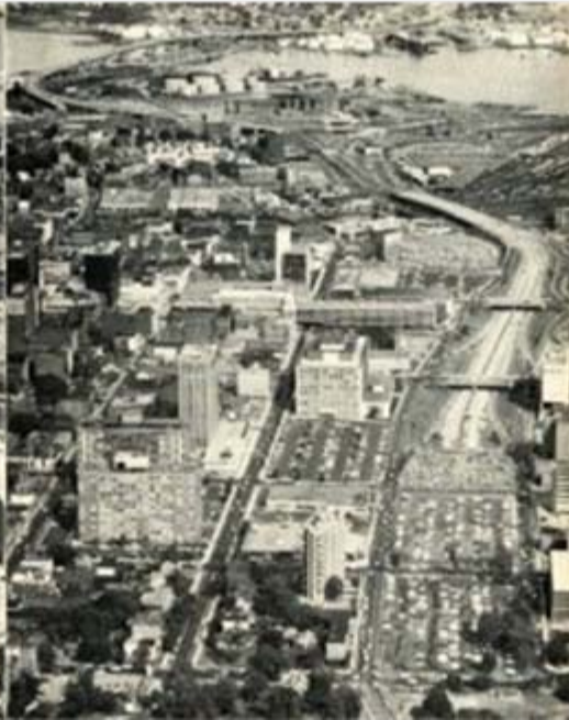
After Route 34 was Built
